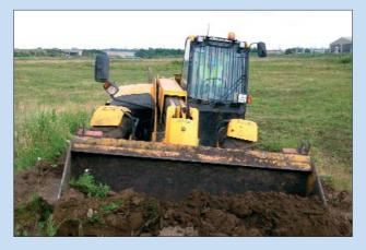
Collecting soil contaminated with polycyclic aromatic hydrocarbons (PAHs) from former steelworks activities that had been stored at the site on impermeable plastic to monitor natural attenuation (degradation under ambient conditions) of PAHs with time. The TWIRLS project used this soil to demonstrate the effect of composting on PAHs.
