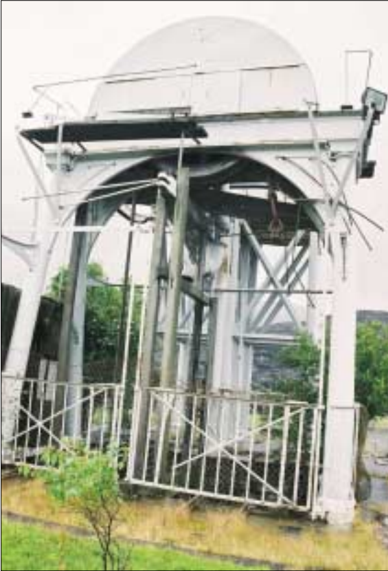
Photo 2. A Victorian water balance lift preserved at Penrhyn Quarry, Wales. The weight of a filled water tank could uphaul a platform carrying slate-laden wagons.
