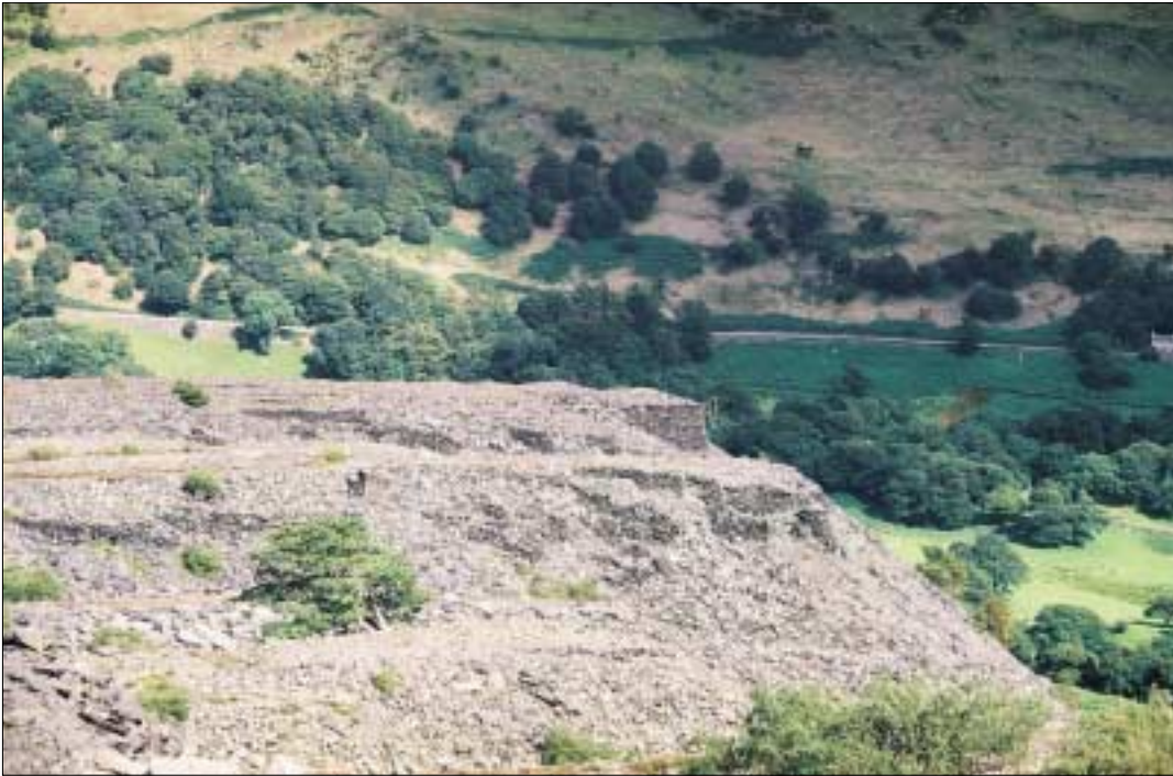
Photo 4. 'Pencilips' are examples of slate waste tips that were once hand-faced along their advancing head, in the late nineteenth century.
